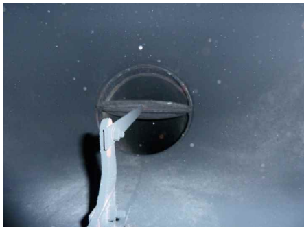
Manually operated damper open and closed
